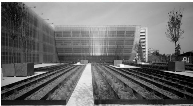
Office building in Pireos Ave.
